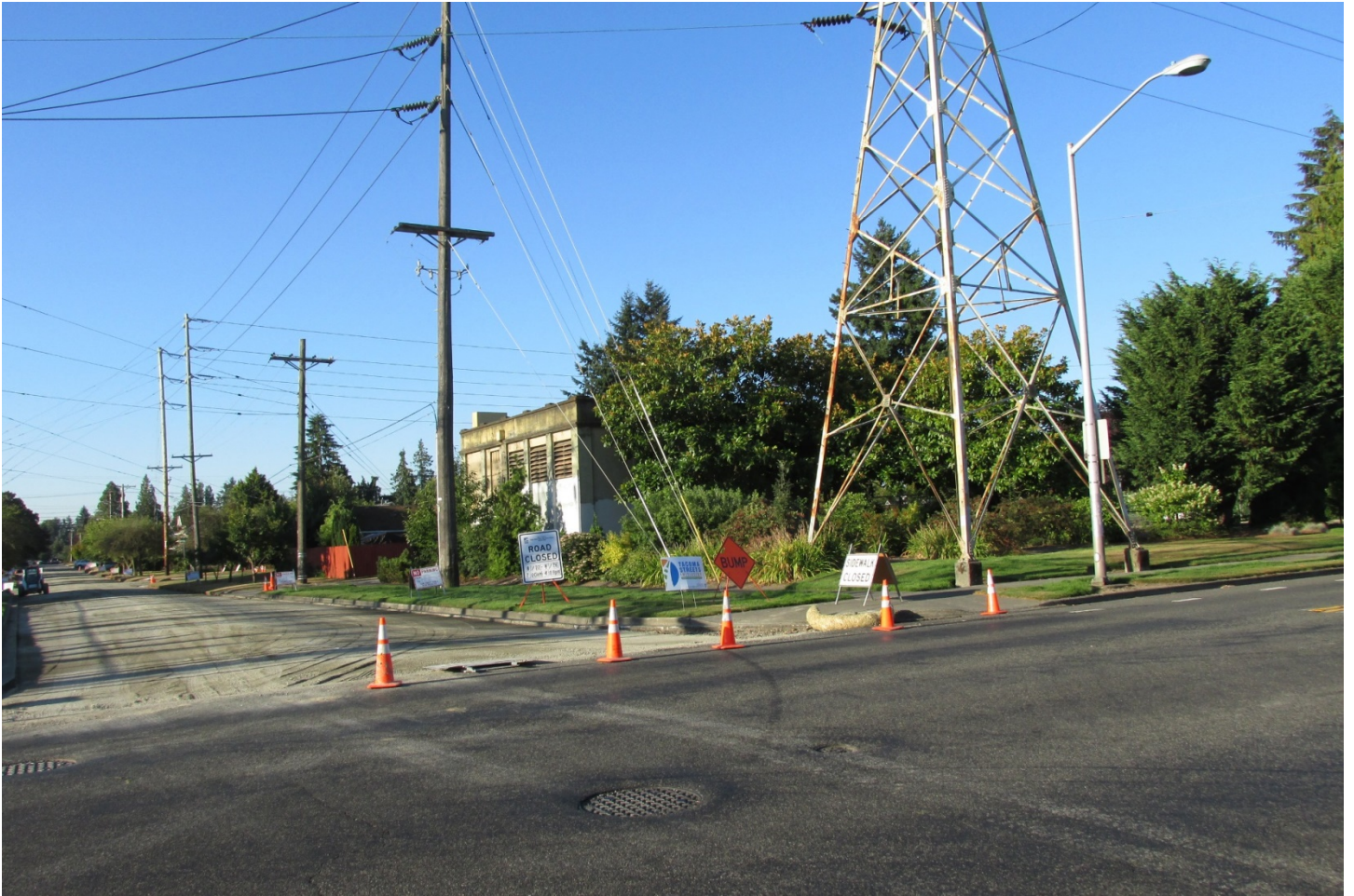
Figure 22 Adams Street Substation and Tower 1, view southwest
