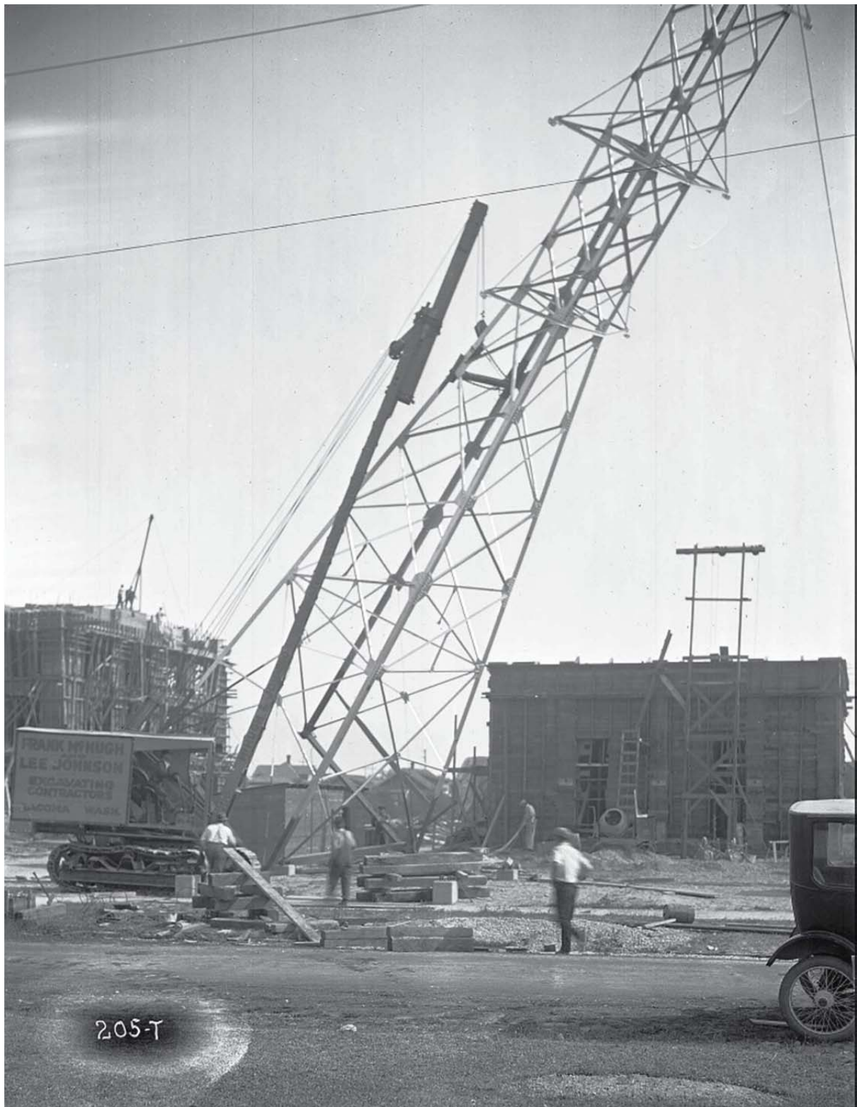
Figure 4 Raising of Tower 1 with Adams and Cushman Substation in background August 4, 1925, Image courtesy of Tacoma Power
