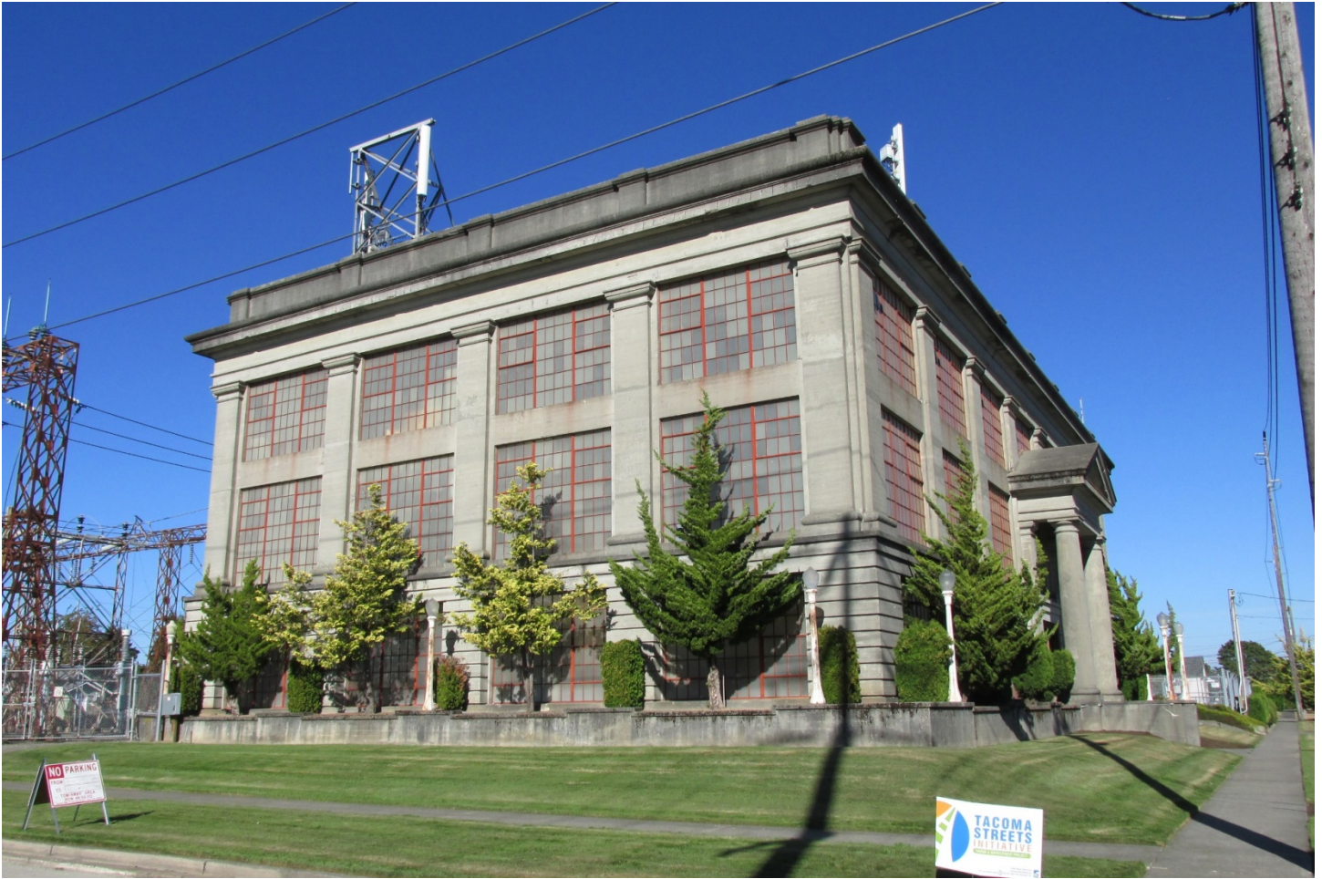
Figure 18 Cushman Substation, view northeast
