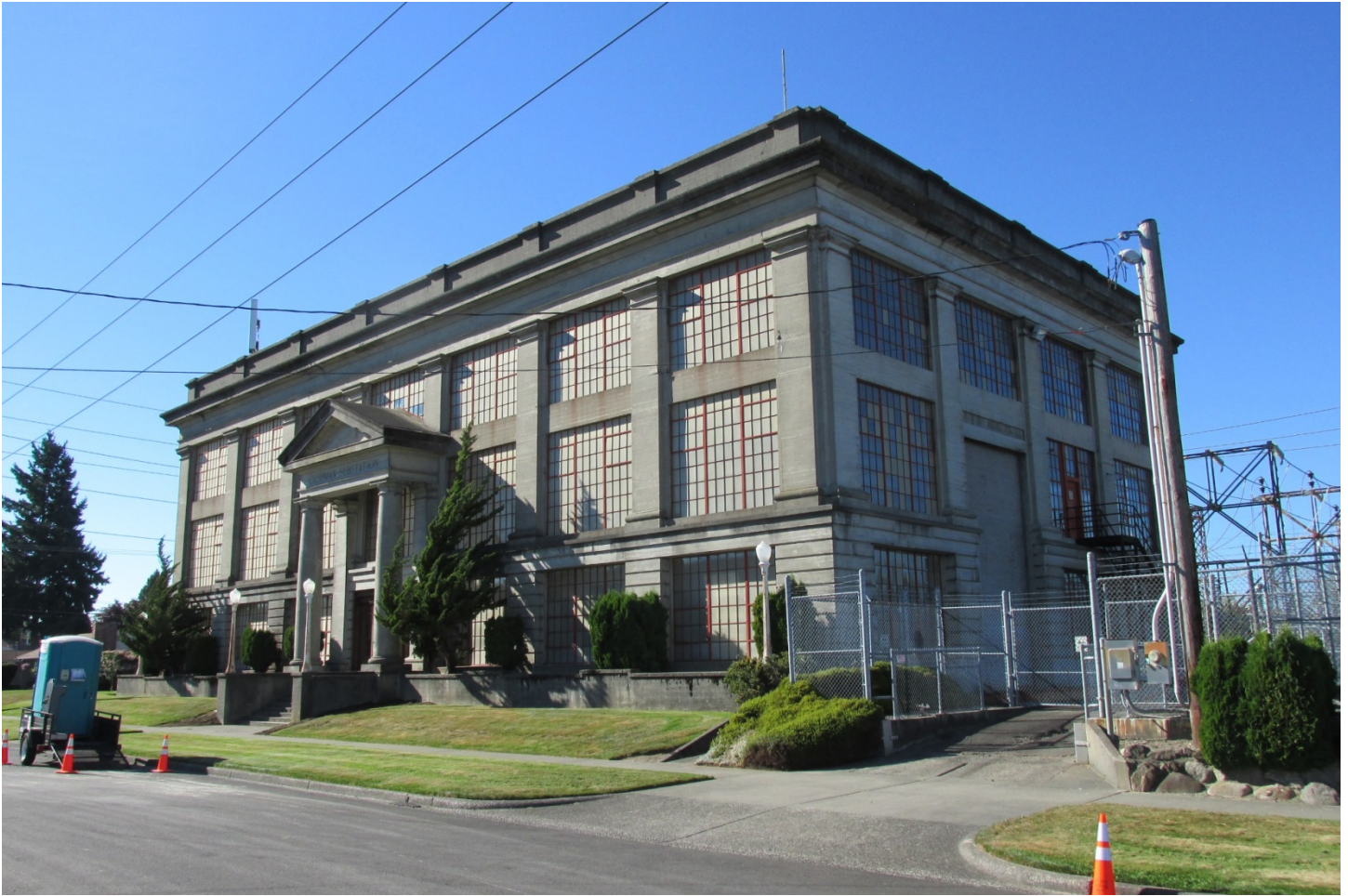
Figure 17 Cushman Substation, view northwest.
