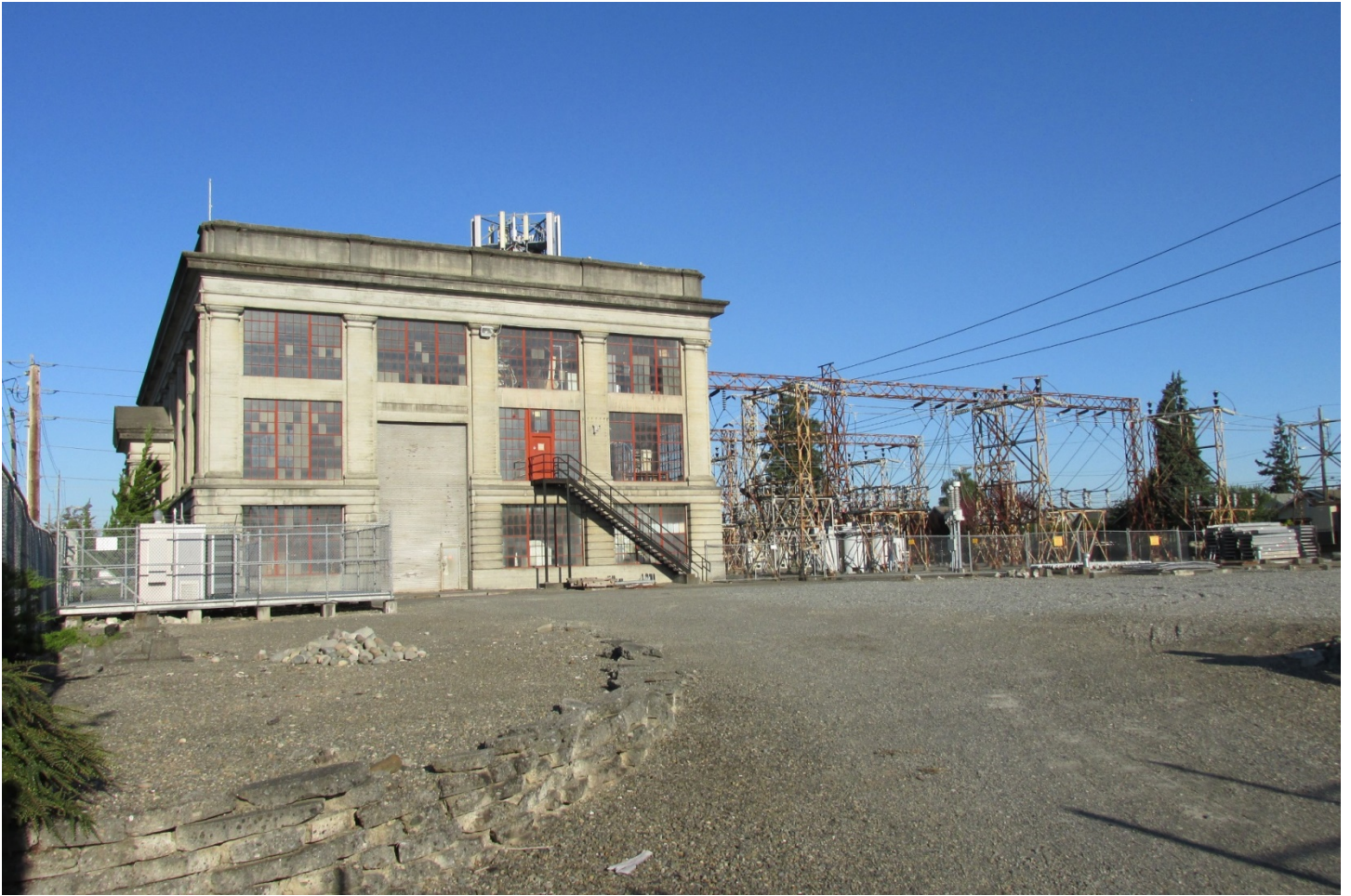
Figure 21 Cushman Substation, view west
